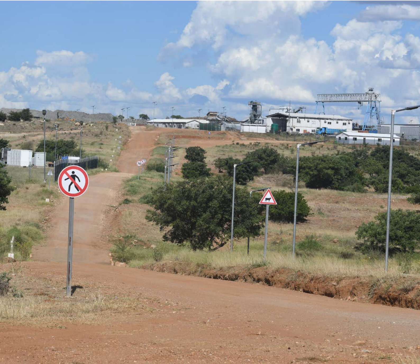
The Road connecting Molo Mine Camp to the Plant Area.
