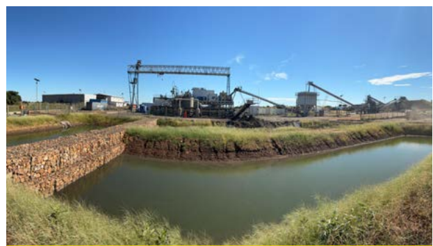
View of the storm and process water control infrastructure.
