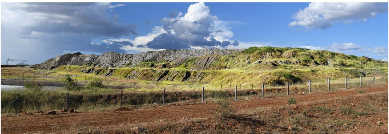
The Molo tailings storage facility showing partially vegetated slopes and access control.
